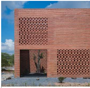
Brise soleil in brick
