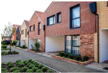
Use of brick to create variety
