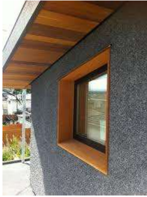
Overhanging roof and deep window reveals
